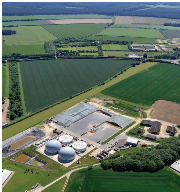
Energy source: 3i-backed biogas producer Future Biogas is working with customers to help them deliver on their own climate goals
